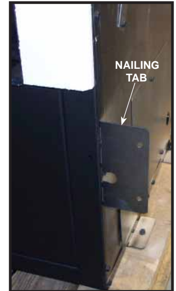
Figure 9.4 Nailing Tabs Installation Position
